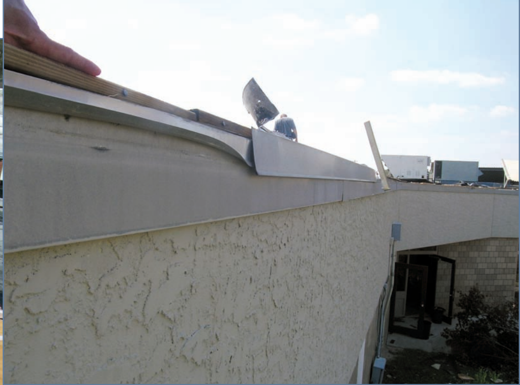
Photo 4: Typical metal edge damage.
