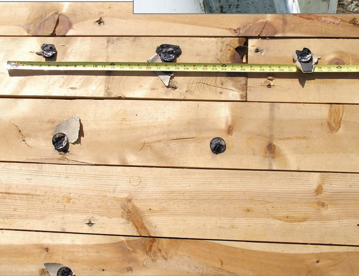
Photo 6: Old BUR attachment. Improper nailing of base sheet did not provide adequate attachment for BUR or new SPF roof system. Side lap nailing is typically 9" O.C.
